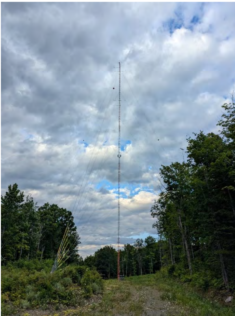
Figure D.3 Mât permanent haubané
